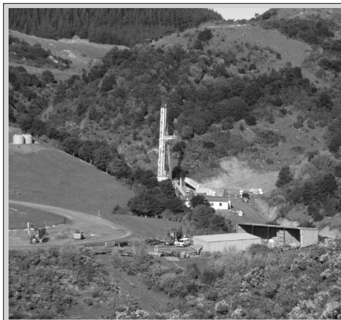
NRG drilling rig at Kate 1 well
