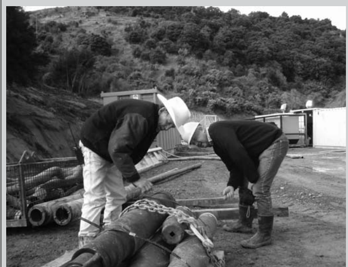
Ron Richards of NRG drilling and Stacey Radford (Green Gate) inspecting drilling equipment.
